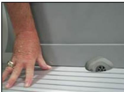
You also need to make sure the edges of the aluminum panels are all lined up. This is necessary to make the installation of the stringers much easier.
